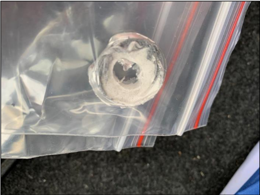
Photograph 4 – Sample of ACP cladding taken from the SW corner of the facade
