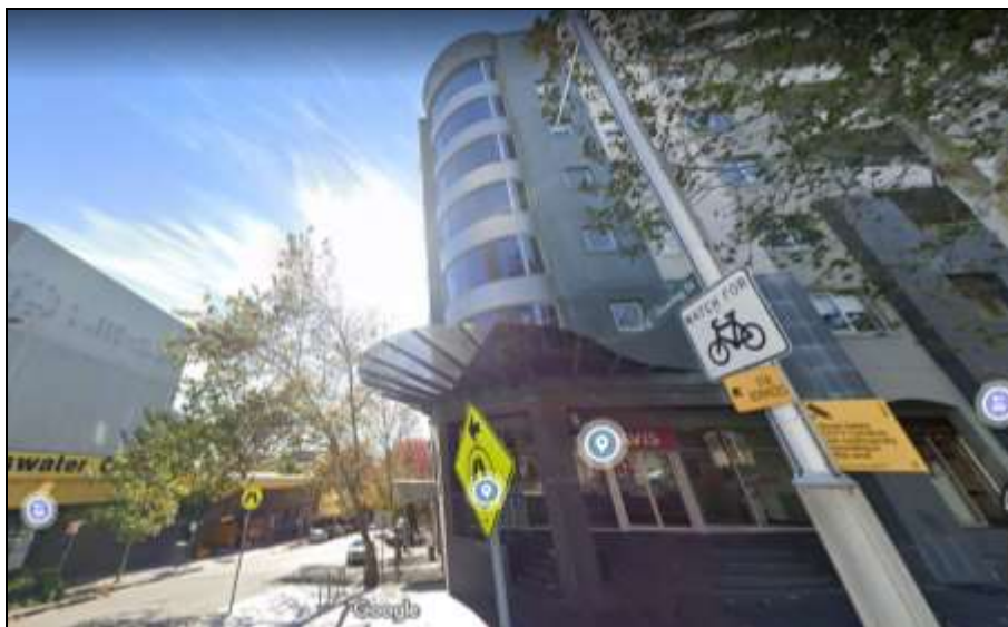
Relationship of the subject site (left) to Marquis apartments (right and opposite) showing glazed areas and light. Source: Google Maps/Streetview
