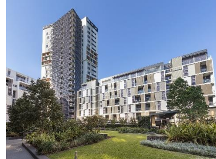
MERITON MOORE PARK PRECINCT Over 2000 Lots / 9 Strata Schemes Retail Precinct, Shared Facilities under BMC
